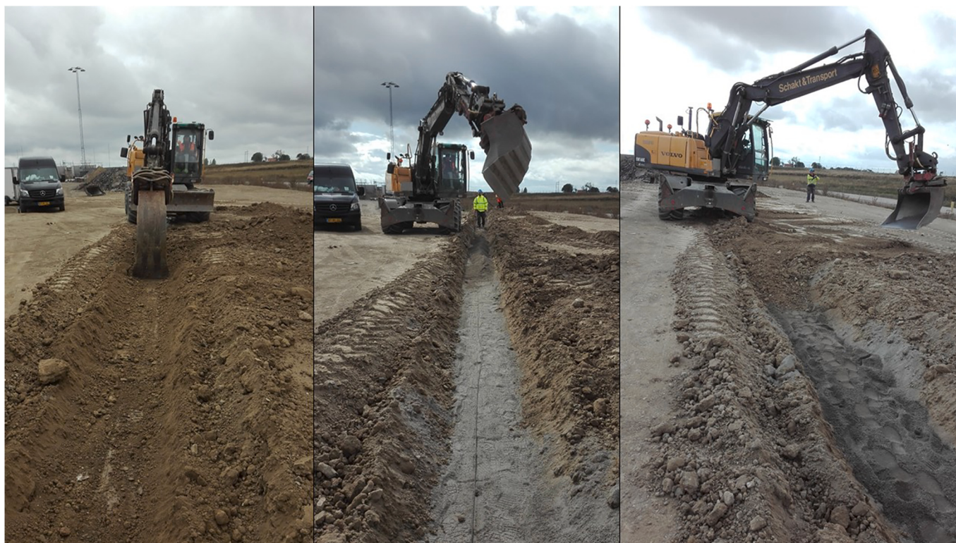
Fig. 3. Pictures of the installation of the fiber optic cable in the ground: left, digging of the trench; middle, cable on top of sand layer; right, backfilling of the ditch with sand and excavated material.
